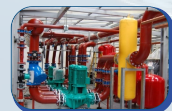
Chilled Water Pump Installation HVAC
