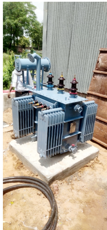
● Transformers Installation & Commissioning
