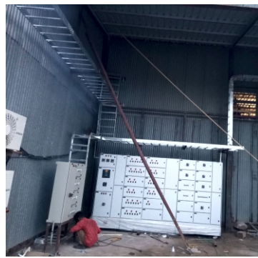
● LT Electrical Panel Installation & Commissioning
